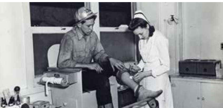
CARE AT WORK: First aid station at Richmond, California, shipyard #3, in 1943.
